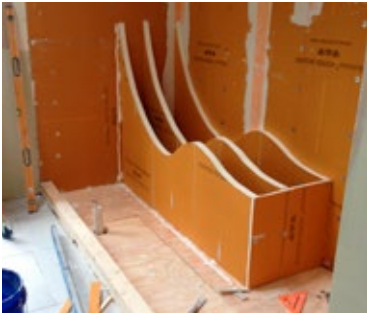
This steam shower included a custom-built chaise lounge inside that needed to be contoured comfortably to the client's height and body type. Blue Tool Box built a full size mock up out of wood that they tailored to the customer's measurements and preferences before crafting the template and building the final bench out of foam.
