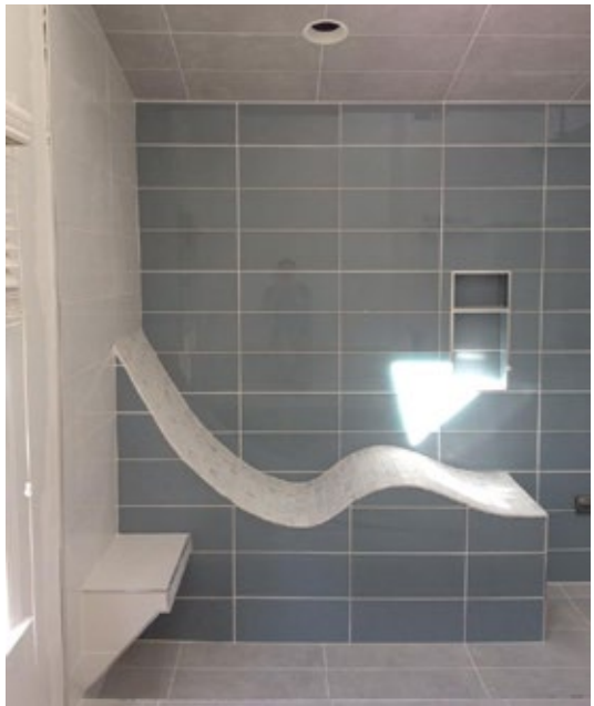
This steam shower included a custom-built chaise lounge inside that needed to be contoured comfortably to the client's height and body type. Blue Tool Box built a full size mock up out of wood that they tailored to the customer's measurements and preferences before crafting the template and building the final bench out of foam.
